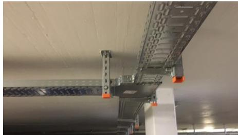
Where so many superlatives come together, OBO is not far away: OBO products from the industrial installation area are also part of the PANDION DOXX project. Vertical ladders and RKSM cable trays will be installed inside the underground car park and across the floors. OBO also convinced the customer with a particular escape route installation with a rail height of 85mm for the entrance to the underground car park.
